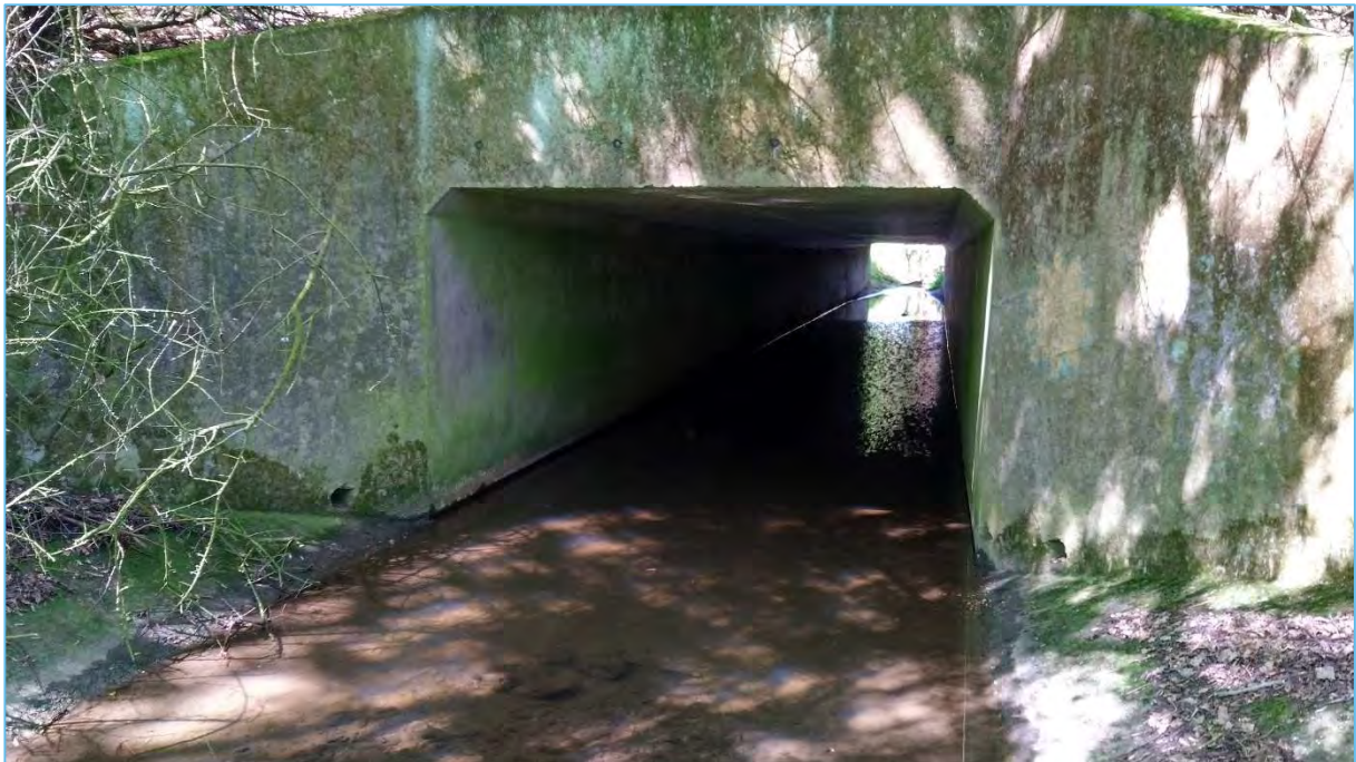
Figure 3.5: Outlet of the 3.0 m x 2.1 m box-culvert under Hall Lane (C11.000)
