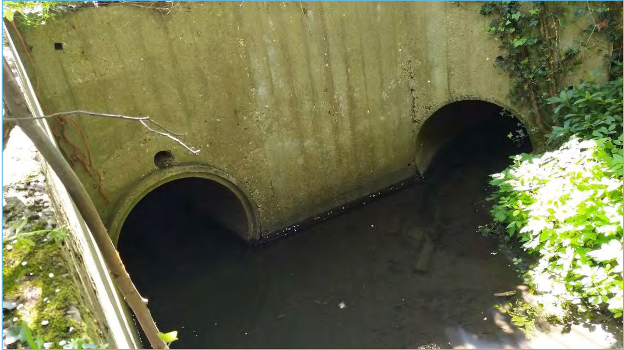
Figure 3.2: Outlets of the \varnothing 900 mm and \varnothing 750 mm culverts under the A1023 (C02.001 and C04.002)
