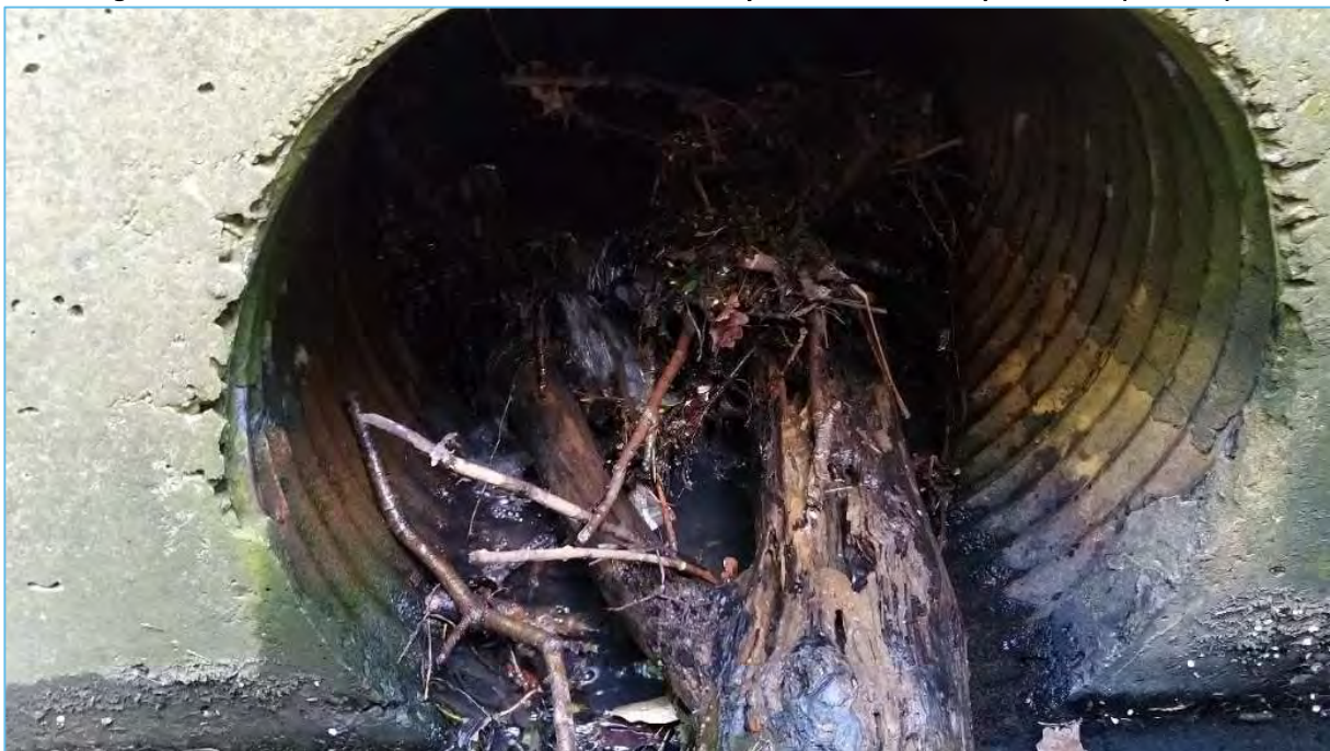
Figure 3.1: Outlet of the Ø800 mm culvert immediately east of the development site (C01.000)
