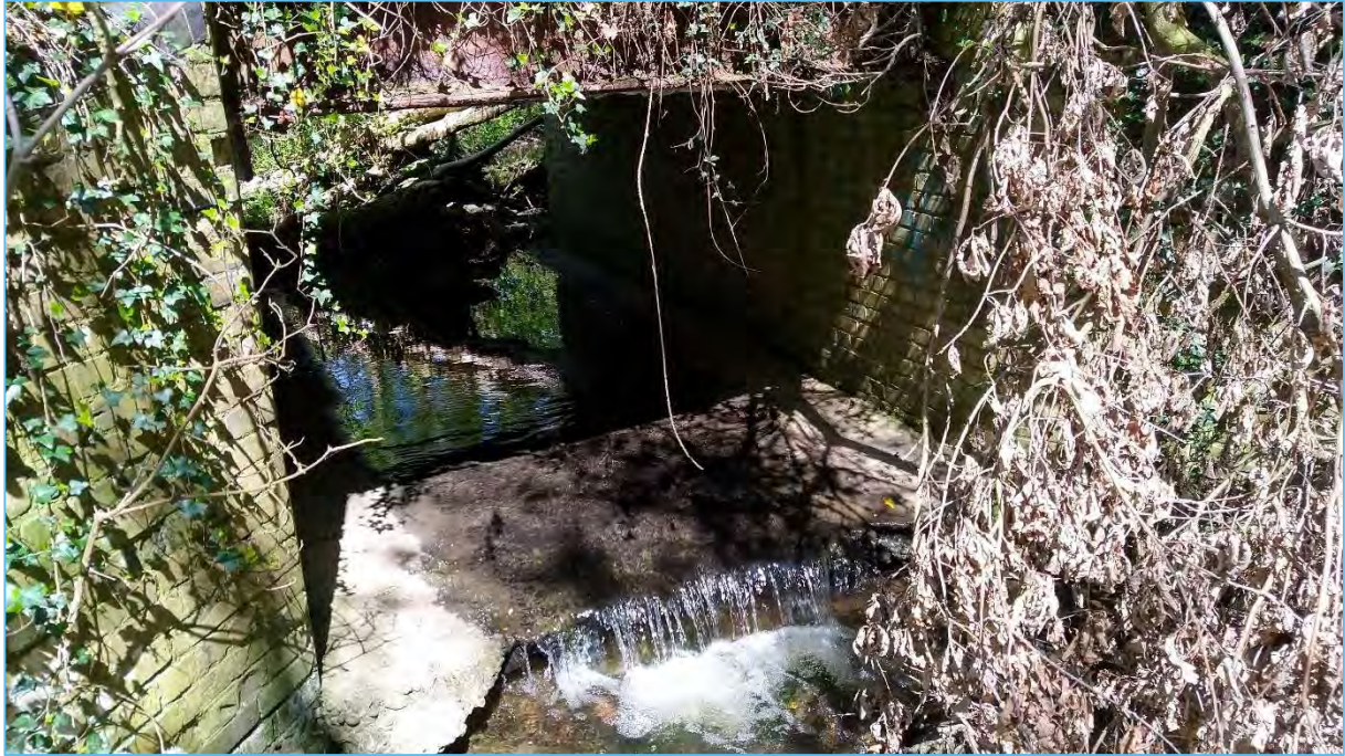
Figure 3.4: Outlet of the 2.4 m x 1.6 m box-culvert under a rural track (C10.000)
