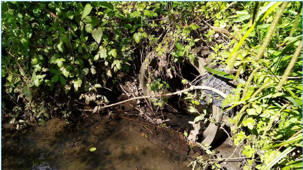
Figure 3.3: Inlet of \varnothing 300 mm culvert under the A1023 (C06.000)
