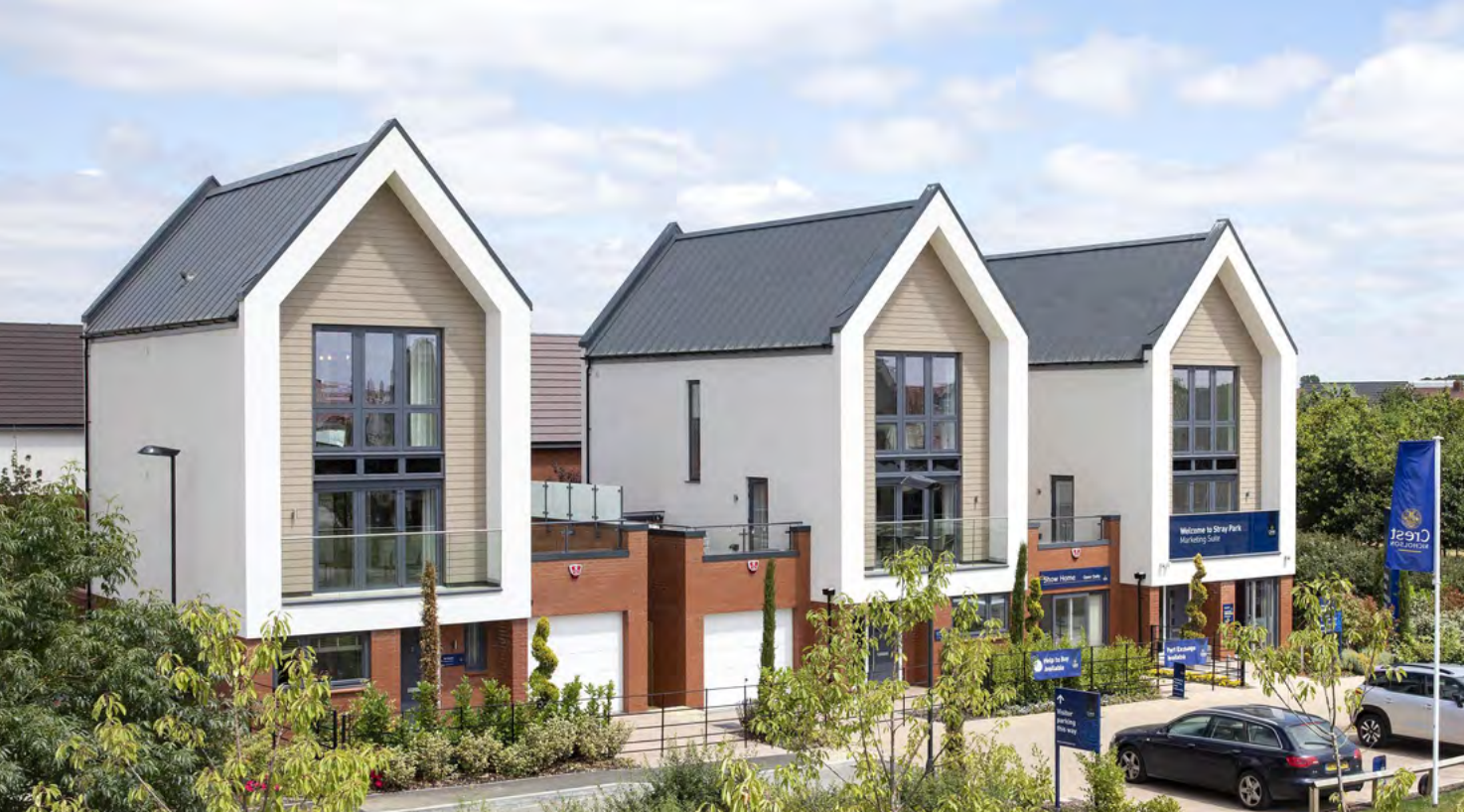
Figure 170. Frontage includes elements of soft landscape, in addition to well-designed hardscape. Tadpole Garden Village, Swindon - Crest Nicholson
