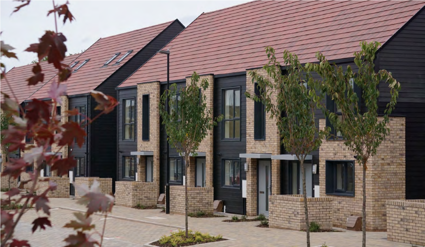
Figure 40. Welcoming and accessible entrances
