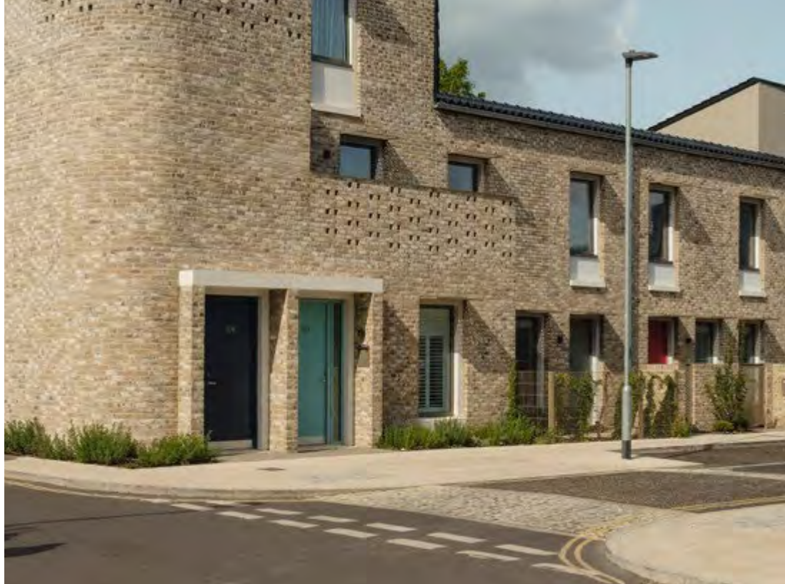
Figure 167. Clearly visible entrances with defined points of entry. Goldsmith Street, Norwich- Mikhail Architects
