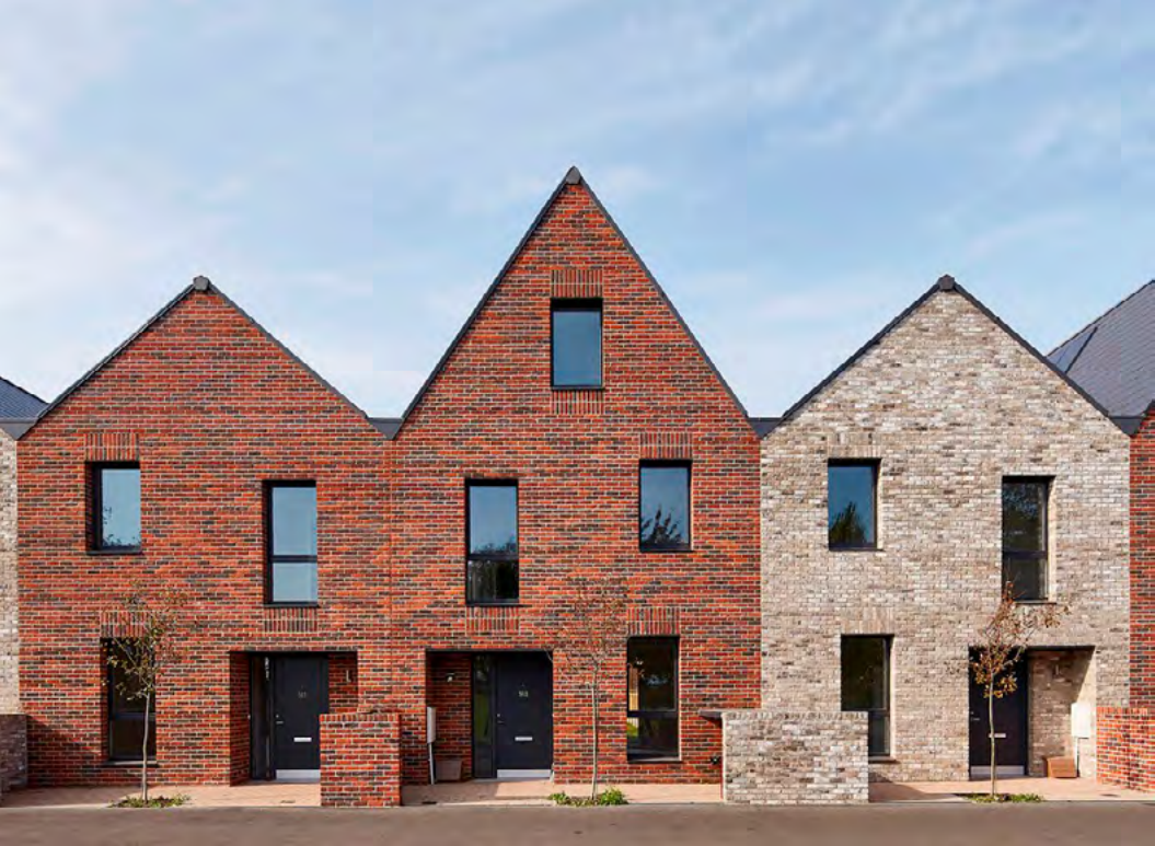
Figure 221. Variations in roof profiles help create variety along the natural setting. St Chads, Tilbury, Essex - Bell Phillips Architects
