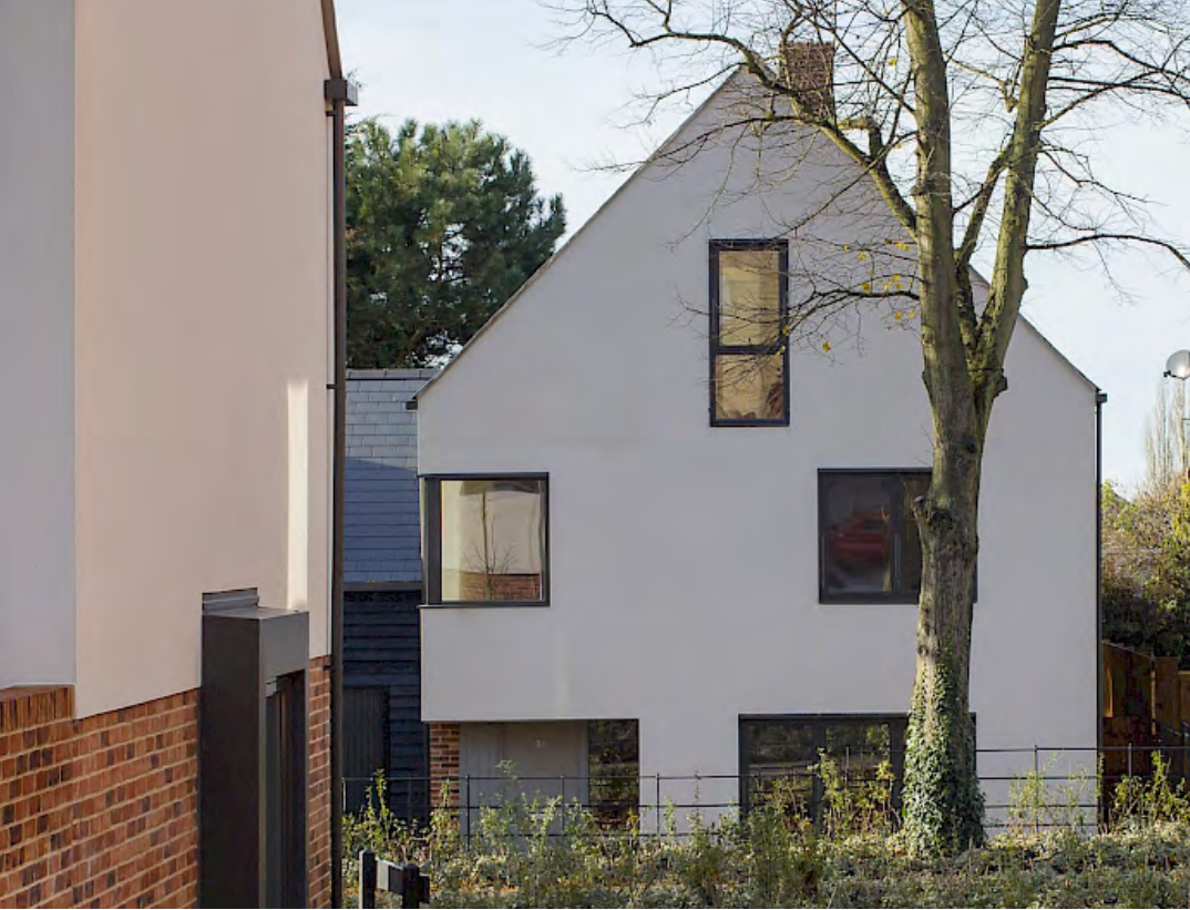
Figure 175. Clear and consistent placement of doors and windows. The Avenue, Saffron Walden, Essex - Pollard Thomas Edwards
