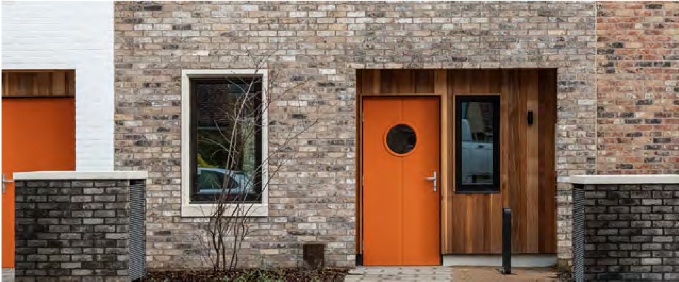
Figure 213. Entrances that reflect the character of Dunton Woods with a prevalence of wooden materials. Marmalade Lane, Cambridge
