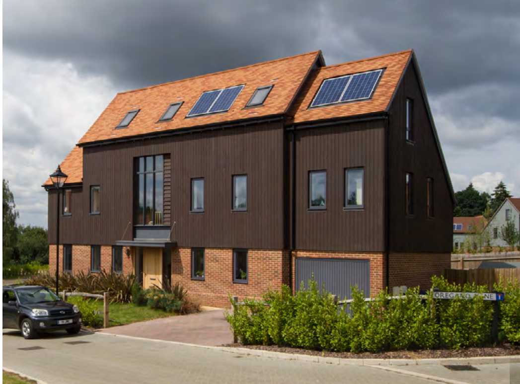
Figure 218. The predominant design articulation should be a feature a datum line, where brick bases are paired with weatherboarding elements for upper floors. Leithfield Park, Surrey - HTA Design
