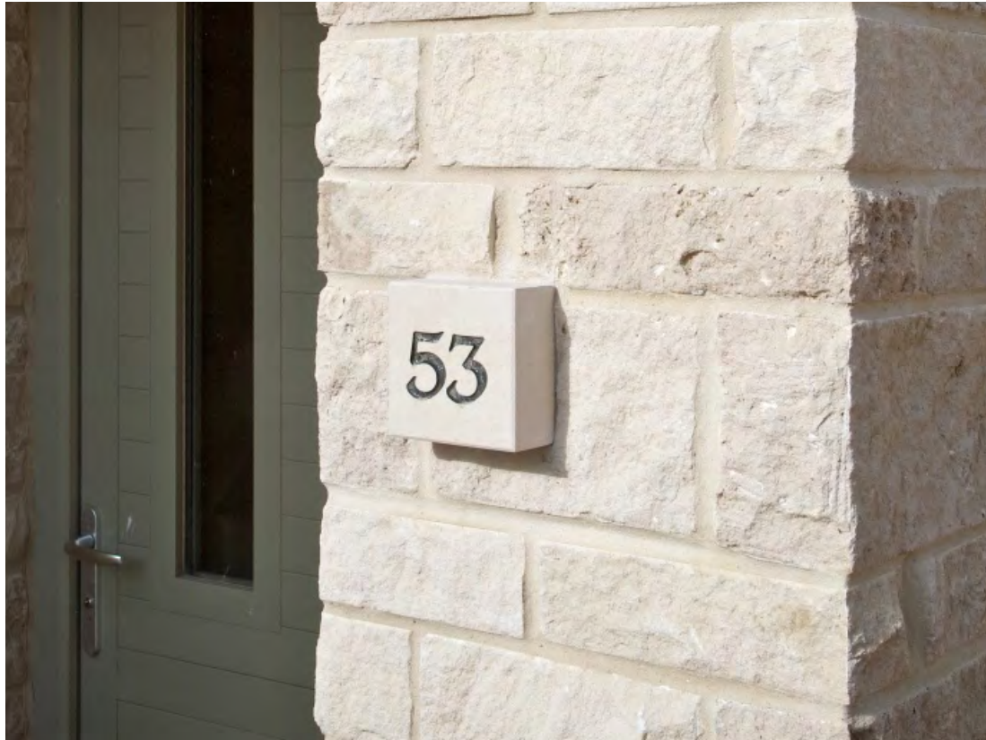
Figure 169. Use of detailing to mark houses. Osprey Quay, HTA Design LLP
