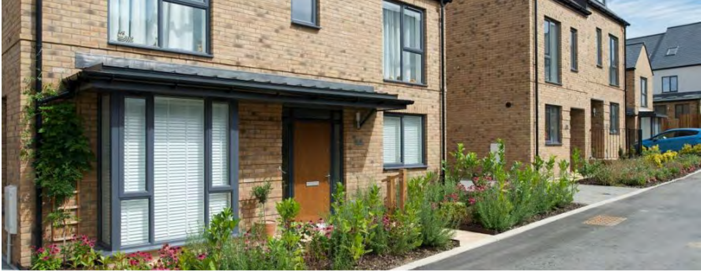
Figure 212. Entrances that are clearly visible with defined points of entry. Cane Hill, Croydon. HTA Design LLP.
