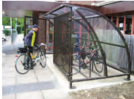
Covered shelter secured with lockable gates
