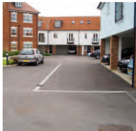
Visible undercroft parking
