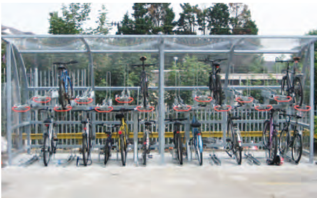
Two tier racks within covered cycle shelter
