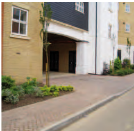
Undercroft secure parking (gated entry).
