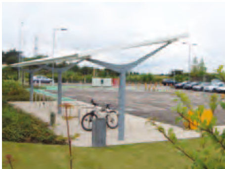
Secure and covered cycle parking at a Park & Ride site
