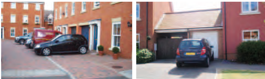
Examples showing the abuse of the 1.5m setback with footway
